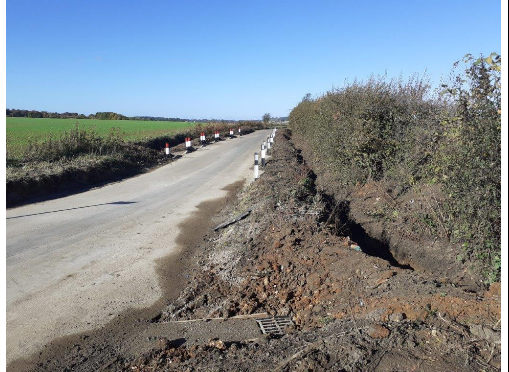
SOAKAWAY INSTALLED & DITCH REGRADE
