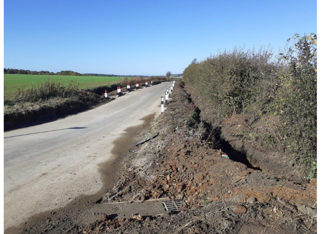
SOAKAWAY, DITCH REGRADE & GRIPS
