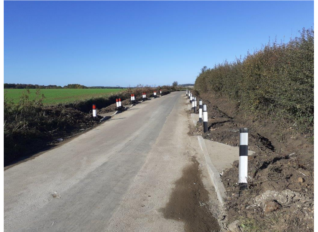
KERBED & CONC. LINED GRIPS INSTALLED ( incl. Verge markers)
