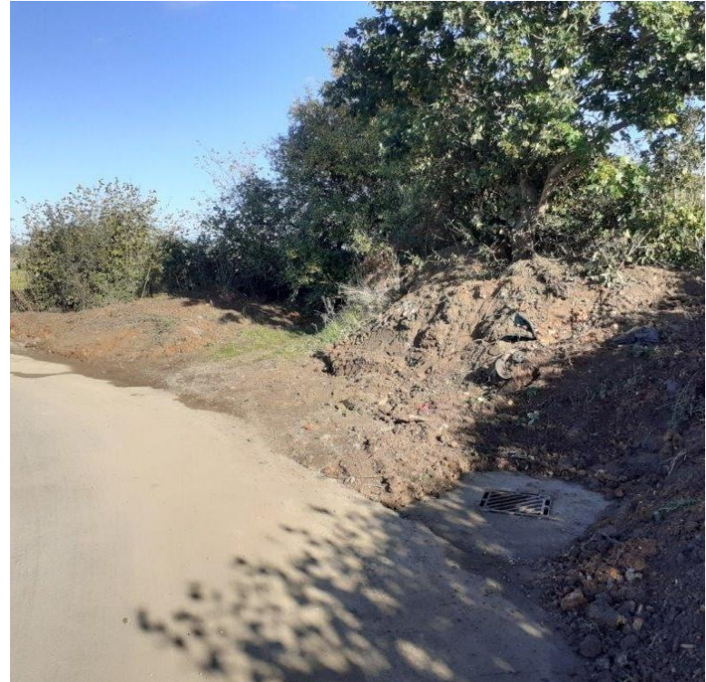
SOAKAWAY INSTALLED
